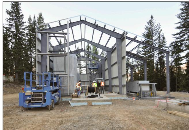
**Construction of energy storage system, enclosure, and controls at Field Substation.**
